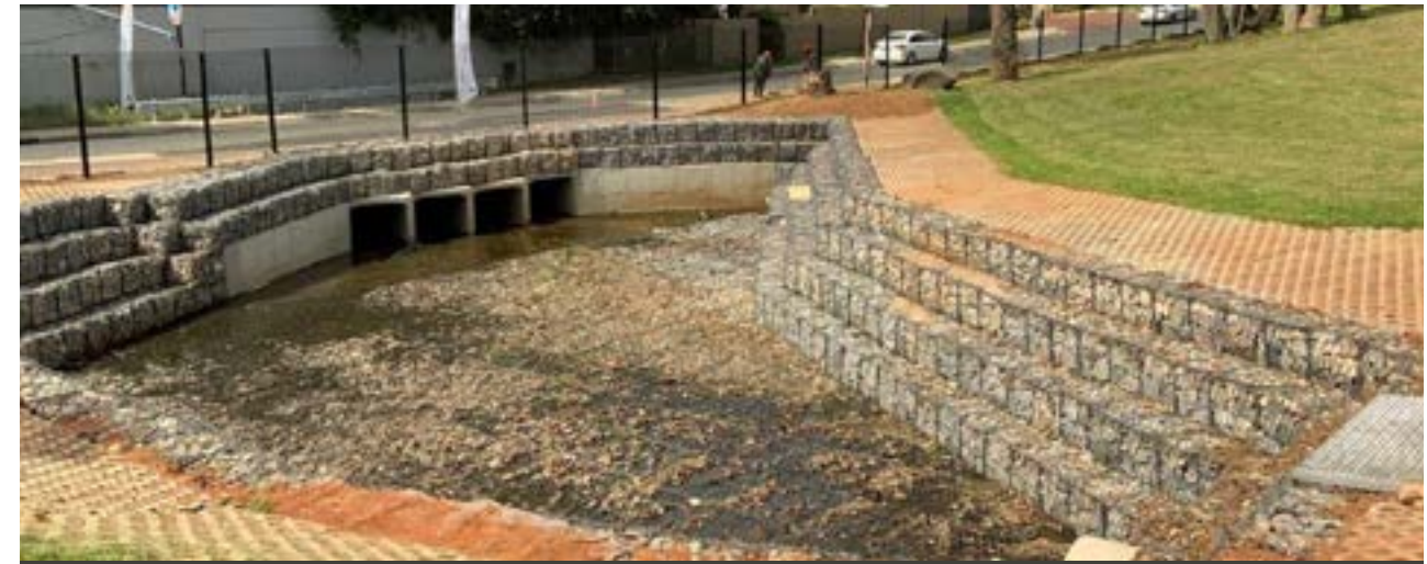
Region E Sandown Mushroom Farm Park stormwater infrastructure rehabilitation
