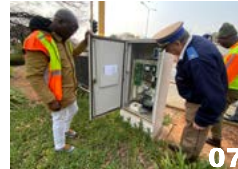
07 The Battle against Theft and Vandalism of Road Infrastructure
