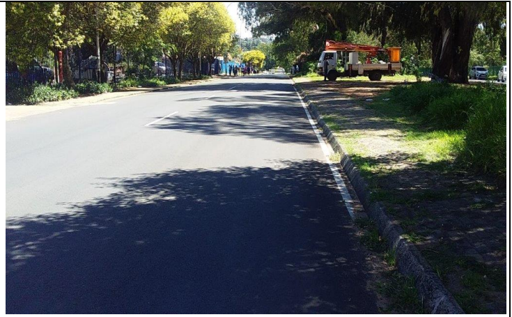
Image 2: Road Resurfaced, Florida, Westlake Road, Region C
