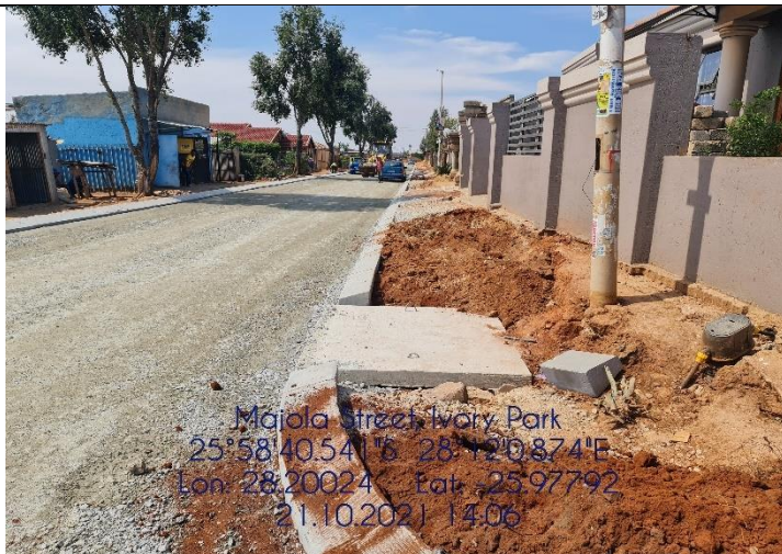
Image 3: Gravel road upgrade-Ivory Park
