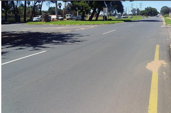
Image 1: Road Resurfaced, Florida, Westlake Road, Region C
