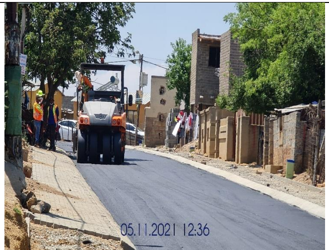
Image 4: Gravel road upgrade- Ivory Park
