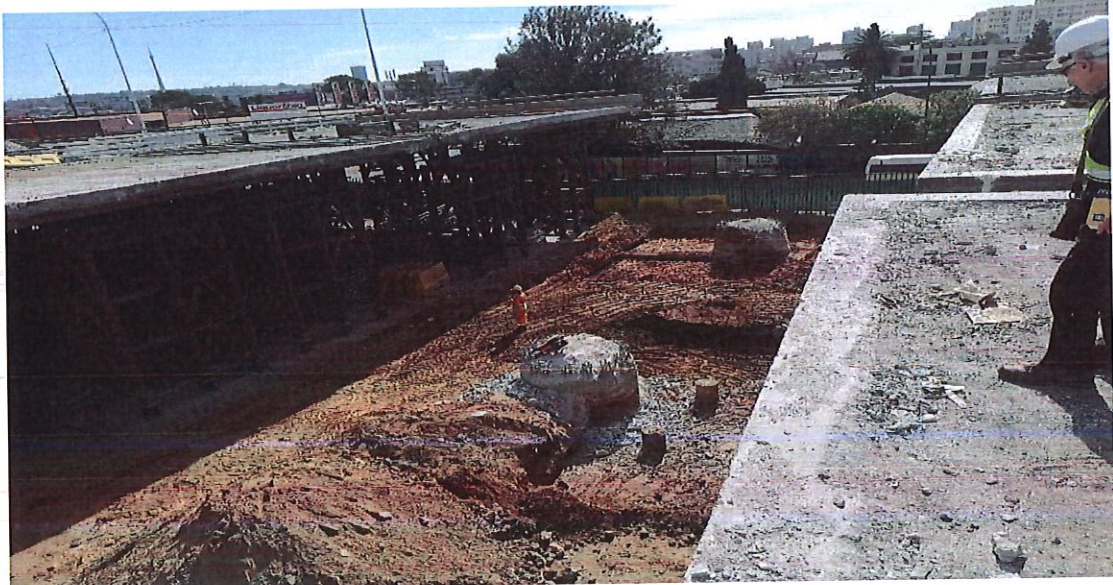
M2 Selby deck demolition
