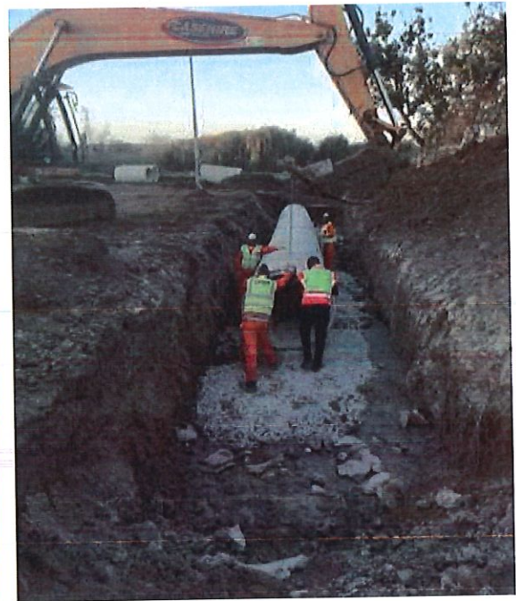
Conversion of Open drains into closed system in Orange Farm and Ivory Park
