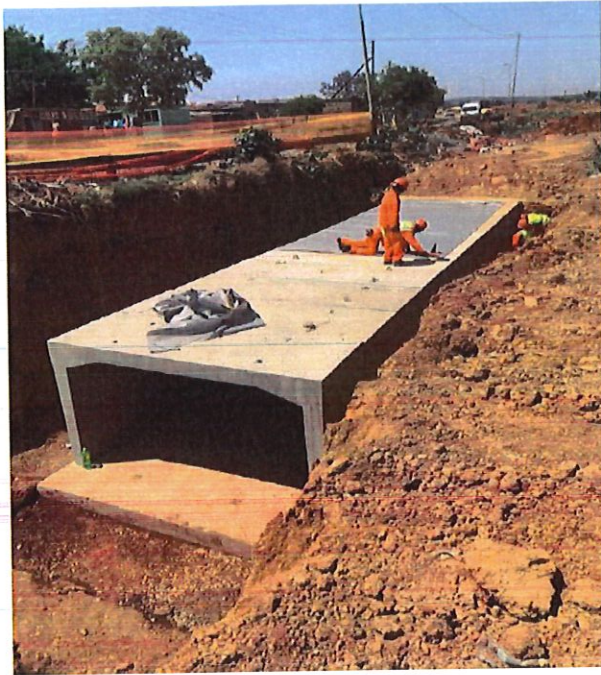
Conversion of Open drains into closed system in Orange Farm and Ivory Park
