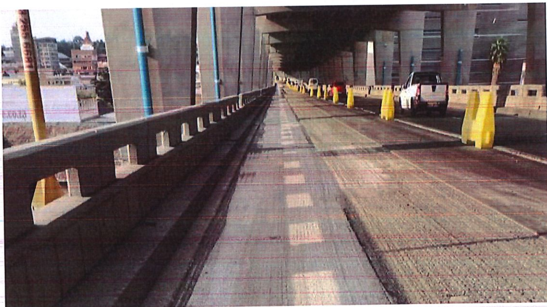
M1 Double Decker rehabilitation
