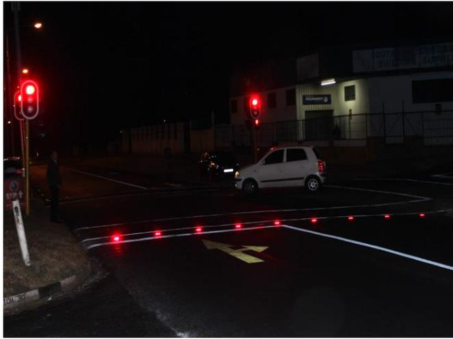
Figure 3 Motorist's view of the LED lane lights
